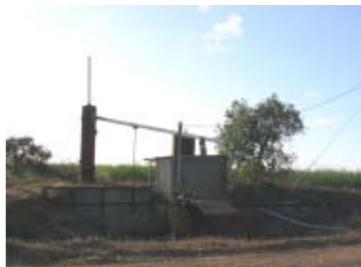
Pumping station between Alva and Ayr (David Scheltinga)
