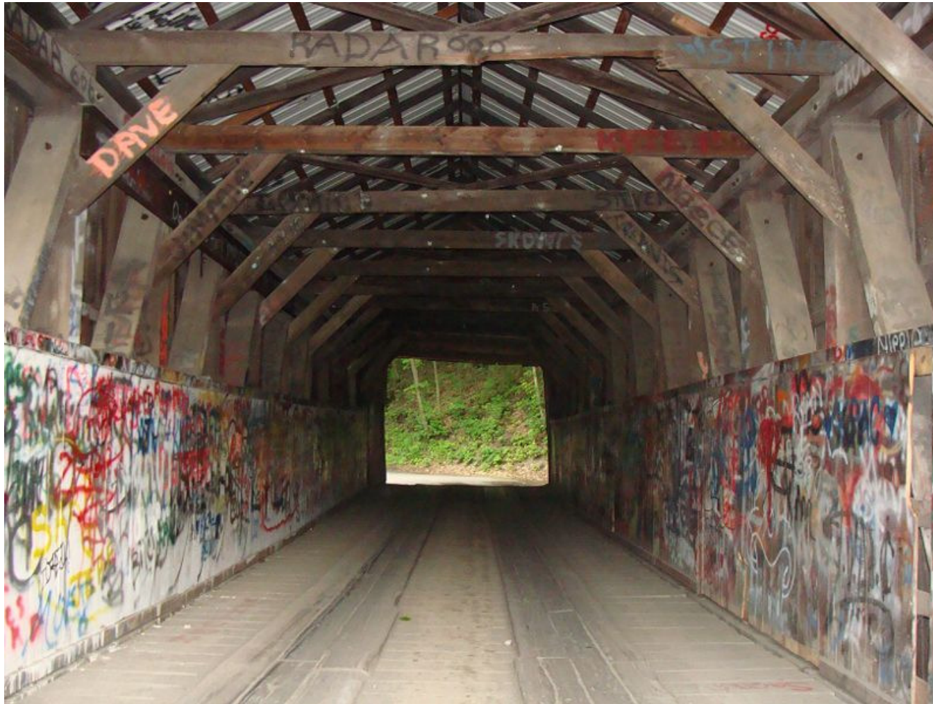
Bridge Interior, with Graffiti July 4, 2008
