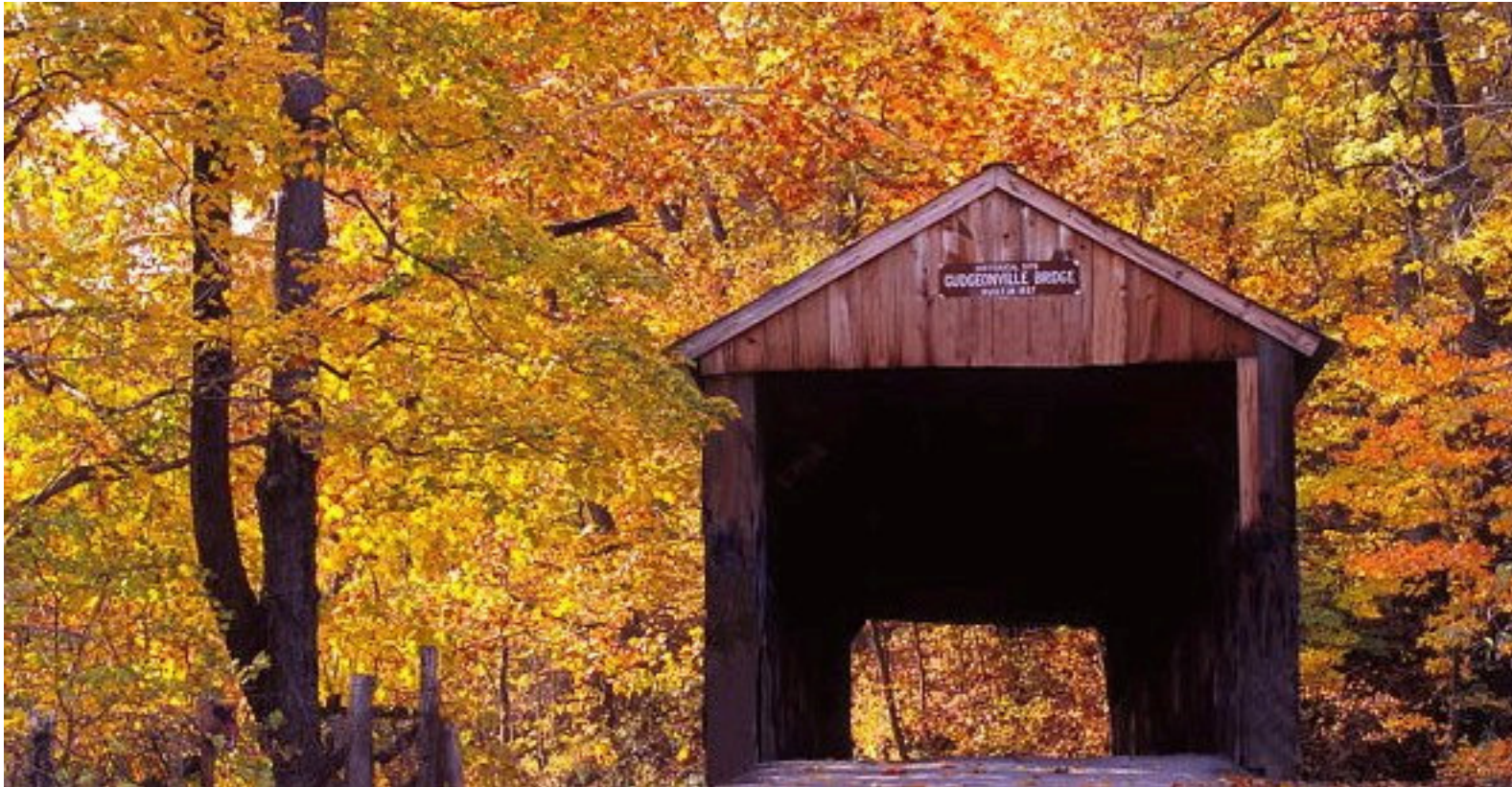
The "Southern" Approach to the bridge, Late October 2005
