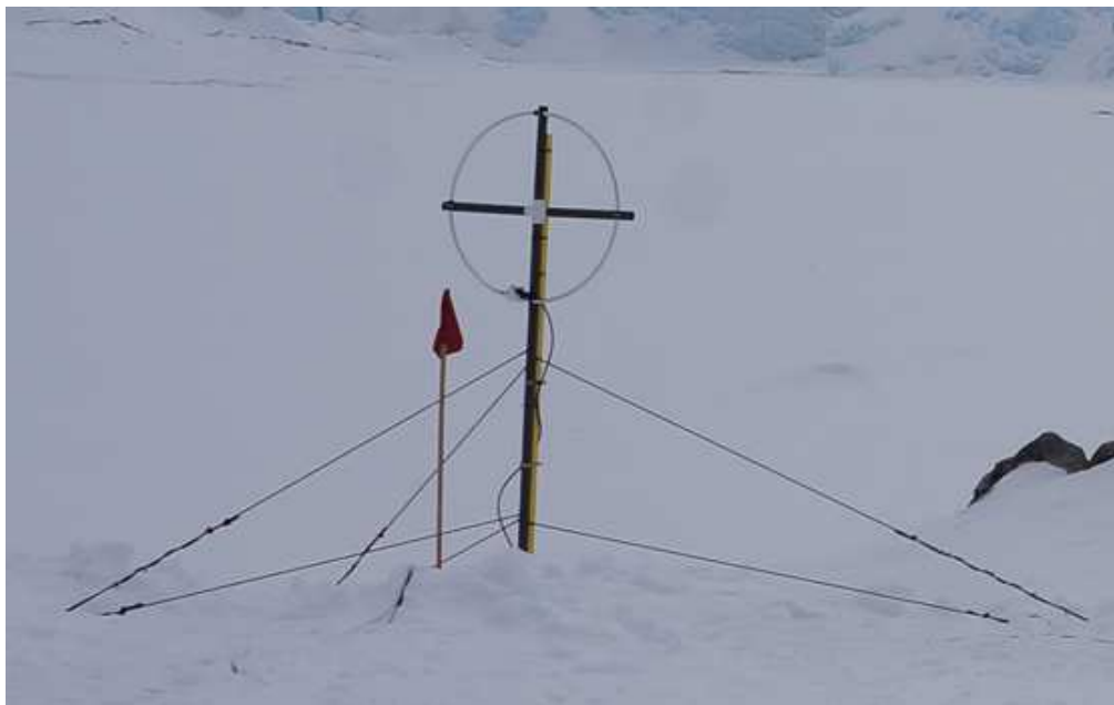
Figure 1. Top: three antenna array installed in Palmer station “backyard”. Distance between the antenna pairs is approximately 25 meters, and antennas are leveled to 1-2 cm accuracy. Bottom: Antenna #2 close-up photo. Yellow reinforcement fiberglass poles were designed, prepared and installed by Joe Bissonnette and Adam Rivers, who also recommended upper and lower guy wires to secure the antenna under high wind conditions.
