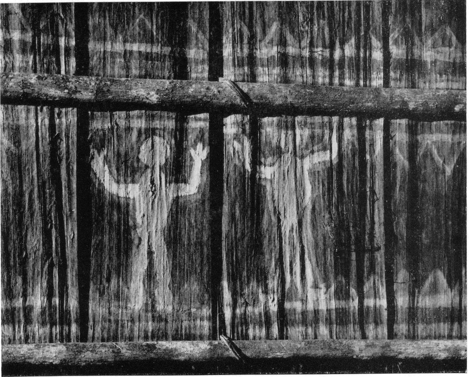
7. Wall of Barasana maloca made of the outer trunk of Socratea exorrhiza , Río Kuduyarí, Vaupés, Colombia.
