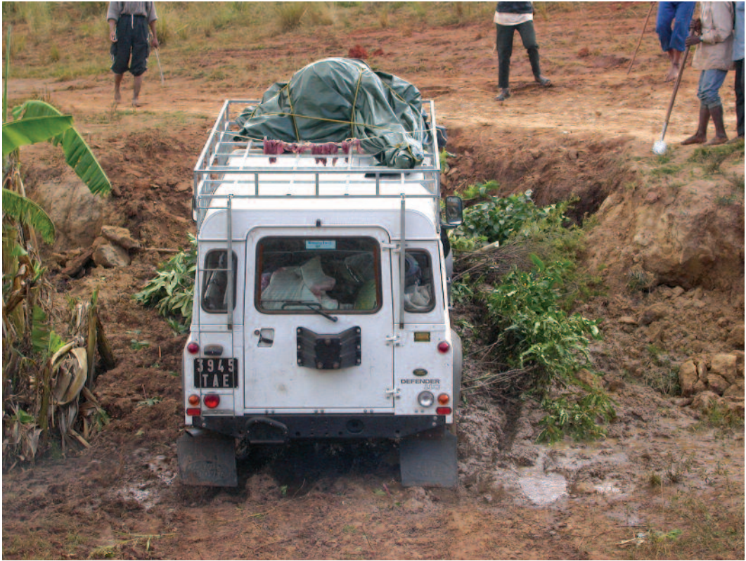
2. Road building on the way to Manalazina.
