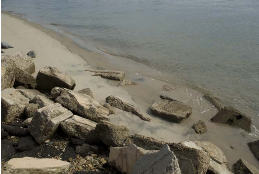
Photo 2-9. Riprap slope in San Diego Bay. Photo courtesy of Rob Wolf.
