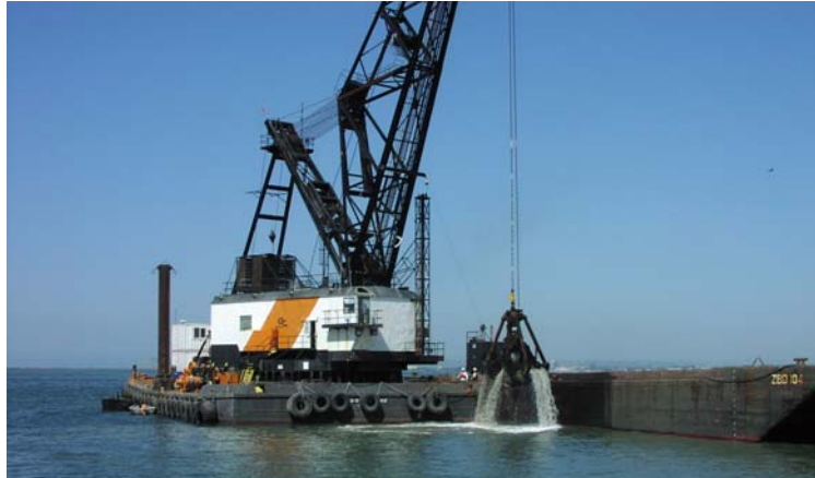
Photo 5-1. Dredging at the wharf. Photo courtesy of Dale Frost.
