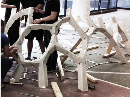
16 Construction sequence occurs in a concentric or row-by-row fashion (Pedersen 2014)
