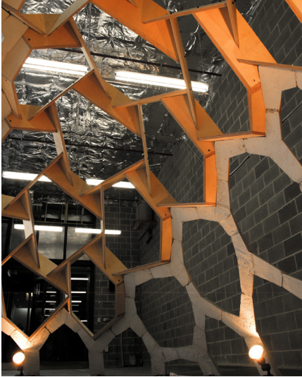
6 Timber Reciprocal Joint Frame (Wibowo 2014)
