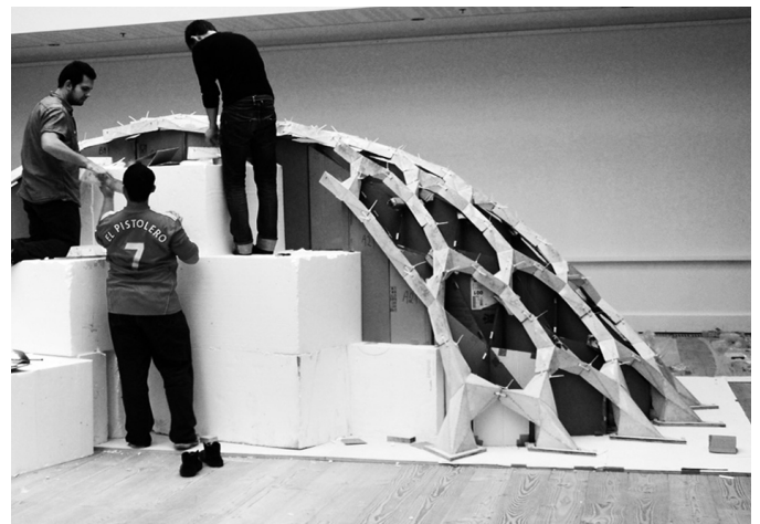
13 The Pre-Vault Pavilion 2012 demanded extensive scaffolding (Pedersen 2012)
