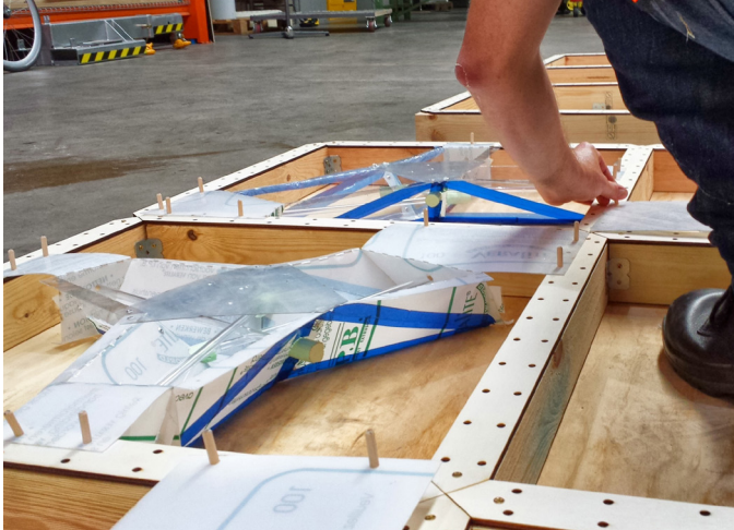
10 Timber casting rigs with alignment dowel holes for increased precision (Bamborough 2014)
