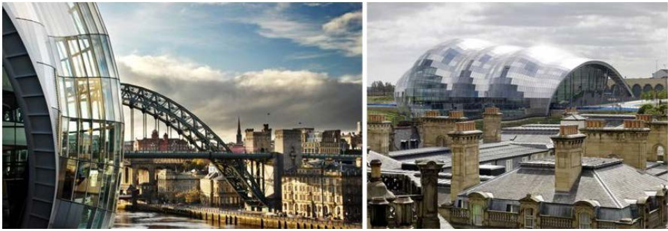
Fig. 4. Foster & Partners, Sage Gateshead, Gateshead, 1998-2004
