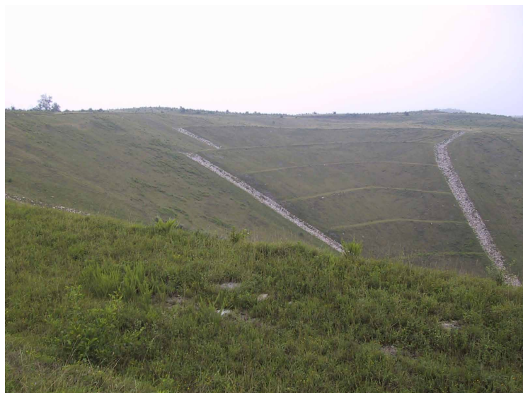
Valley fills can be hundreds of hectares in size. Riprap channels along the sides of valley fills and in streams below the fills channel surface water to reduce erosion. Creation of valley fills buries valuable streamside habitat for semi-aquatic salamanders. Photo: John Edwards, West Virginia University.
