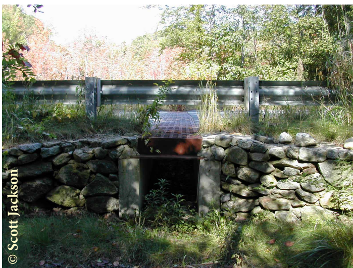
Tunnel for Spotted Salamanders in Princeton, MA. Note the grated top to allow rain to keep the inside of the tunnel wet during migration.
