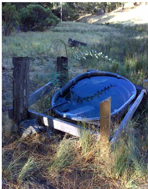
Aquatic escape ramp installed within an existing water trough. Photo by John Meriwether.
