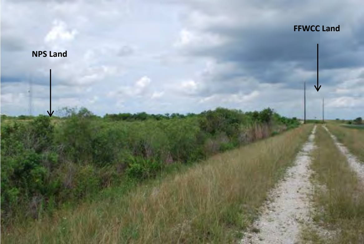
FIGURE 30: EXISTING VIEW NORTHWARD ON L-31N CANAL AVENUE AT EASTERN EDGE OF NPS LAND
