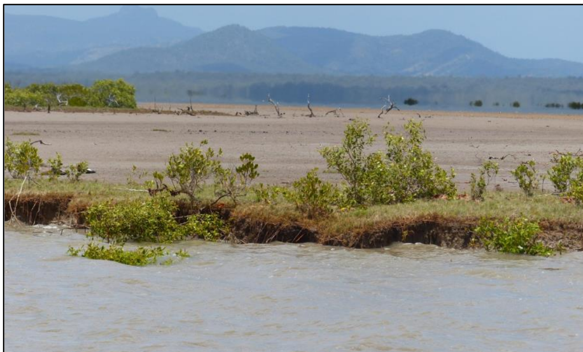
Figure 5.10: Eroded bank in the Narrows, Balaclava Island study area
