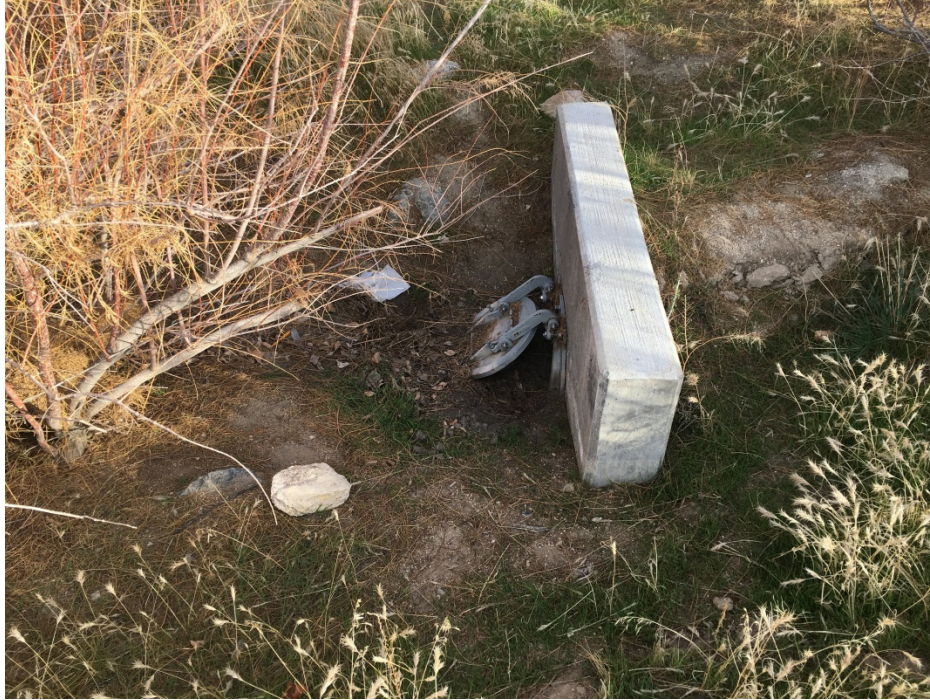
Photo 7. Typical flapgate culvert (ED-03)
