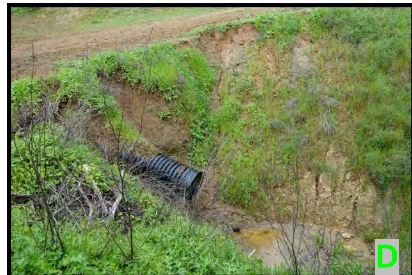
Figure B3: Incision and erosion of road and downstream of culverts, Coyote Canyon, Santa Clara County, CA The location of each photo (A-D) can be seen in Figure B5.
