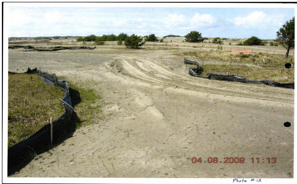
Figure 9. Photo from 2008 investigation report by the U.S. Army Corps of Engineers documenting impacts to the site by the golf course development, including wheel tracks, wetland fill, extensive scouring and sand moving, and tree cutting (USACE 2008).
