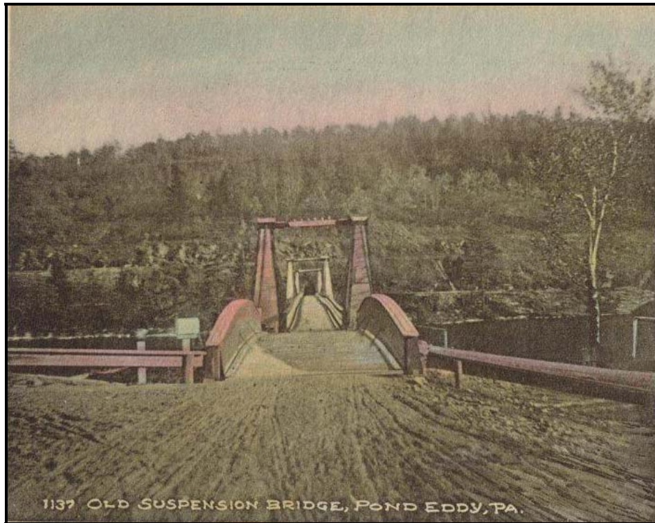
Historic Photo 2. An undated and colorized postcard of the 1871 Pond Eddy Bridge. Postcard courtesy of the Sullivan County (New York) Historical Society
