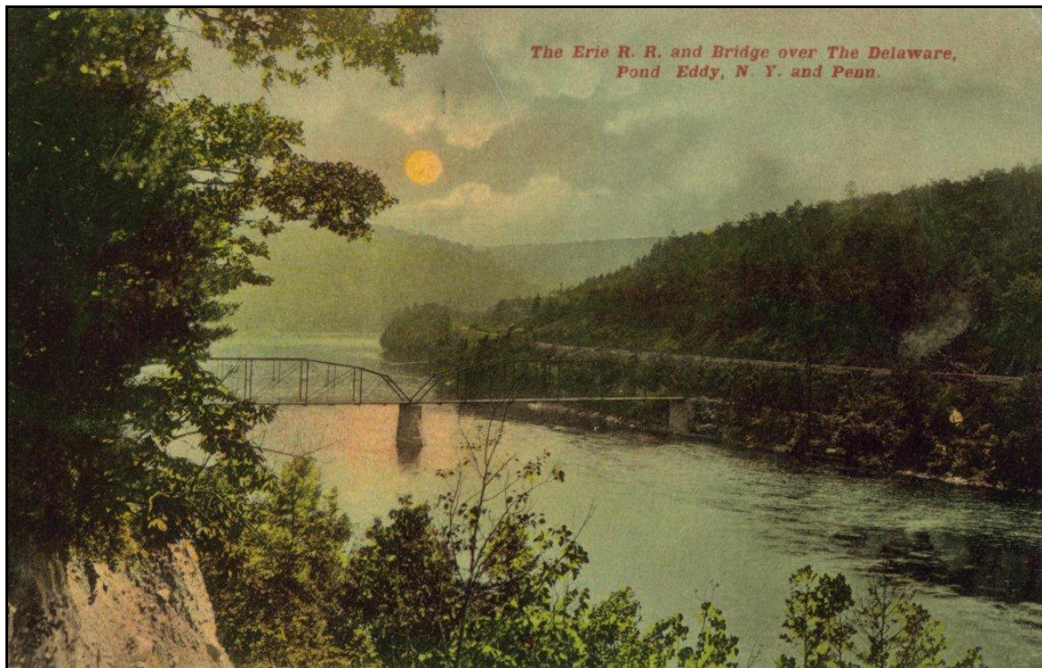
Historic Photo 7. An early twentieth century view looking southeast of the Pond Eddy Bridge and the Erie Railroad on the Pennsylvania side of the Delaware River. Postcard courtesy of the Sullivan County Historical Society.
