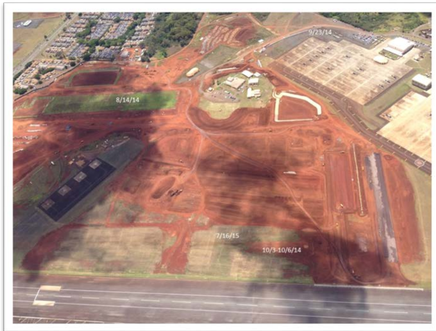
Aerial photo of the WAAF construction site.
