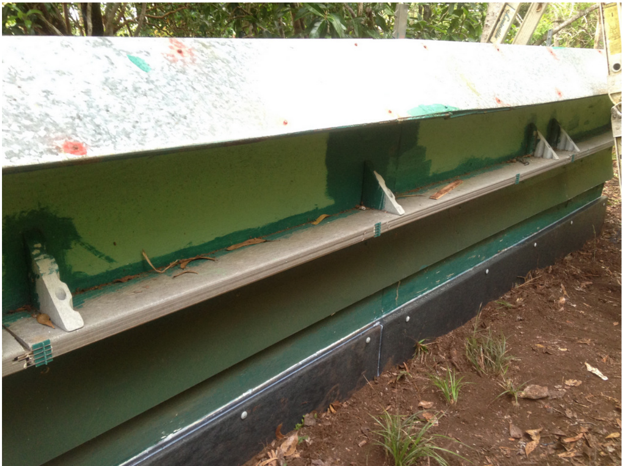
Figure 3. Recent enclosure wall upgrades showing plastic lumber at ground level and wall supports on the inside.
