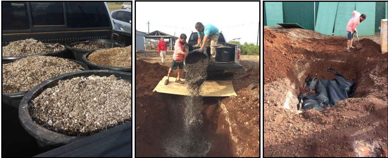
Left to right: contaminated media drying in pots; dumping media into West Base pit; weed mat covering media.
