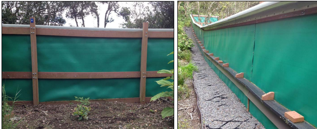
Figure 5. Palikea North enclosure design: wall frame inside of enclosure (left), and outside wall with E. rosea barrier, rat hood, and erosion control (right).
