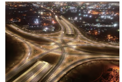
Overpass for an intersection on the main road in Ghana
