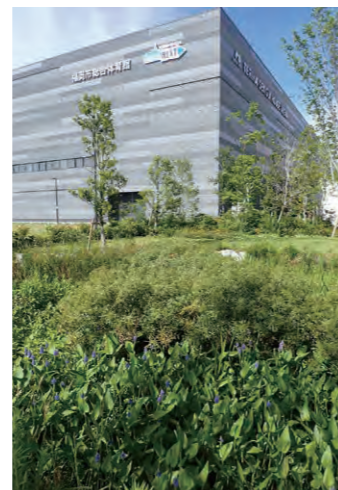
Rain garden in the TERIHA SEKISUI HOUSE ARENA in Fukuoka City
