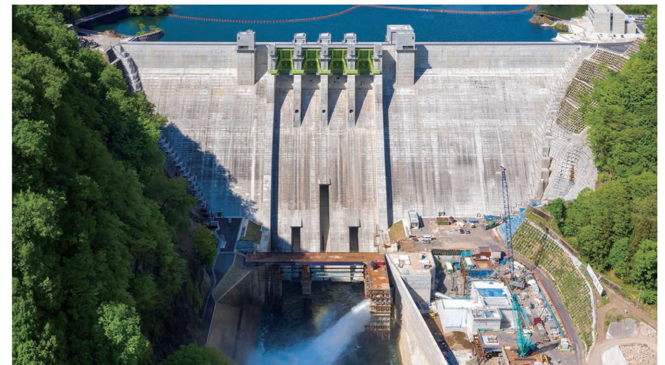
Yamba Dam, a 116-m-high concrete gravity dam (Agatsuma-gun, Gunma Prefecture)
