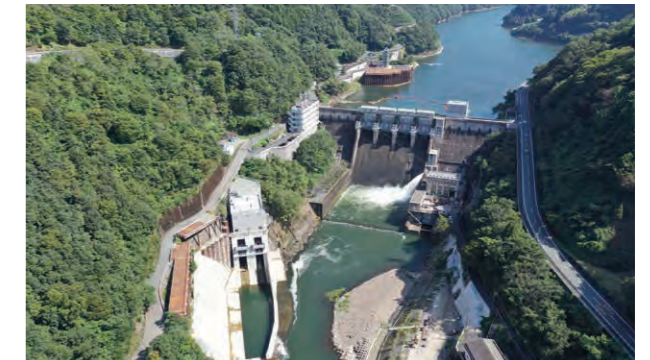
Tunnel spillway (on left in photo) built in the Kanogawa Dam (Ozu City, Ehime Prefecture)
