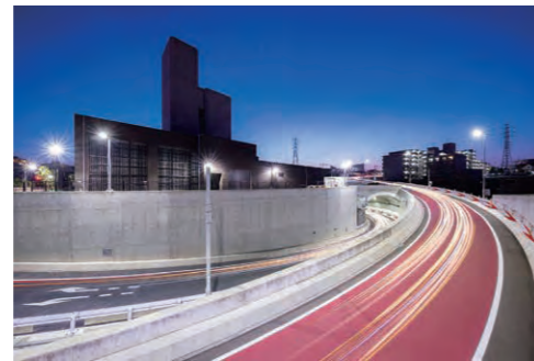
Construction of shield tunnel with a large cross-section in an urban area with steep inclines, sharp curves, and little ground covering (Baba entrance/exit on the Yokohama Expressway North Route)
