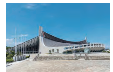
Yoyogi 1st Gymnasium (Shibuya-ku, Tokyo) (First built in 1964, seismic retrofitting completed in 2020)
