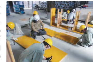
Experience in assembling formwork frames in a hands-on experiential tour for technical high school students
