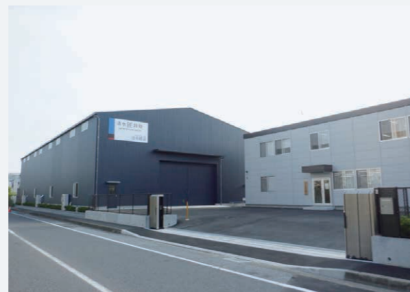
Exterior view of the Shimizu Takumi Training Center
