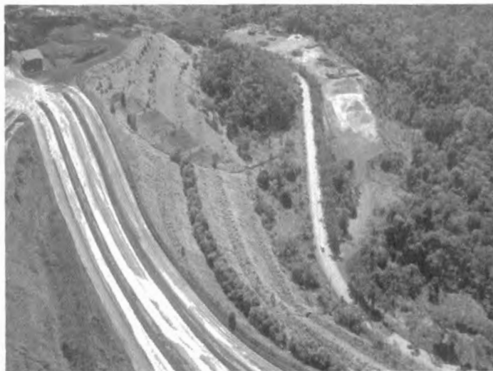
Ongoing rehabilitation of degraded areas.
