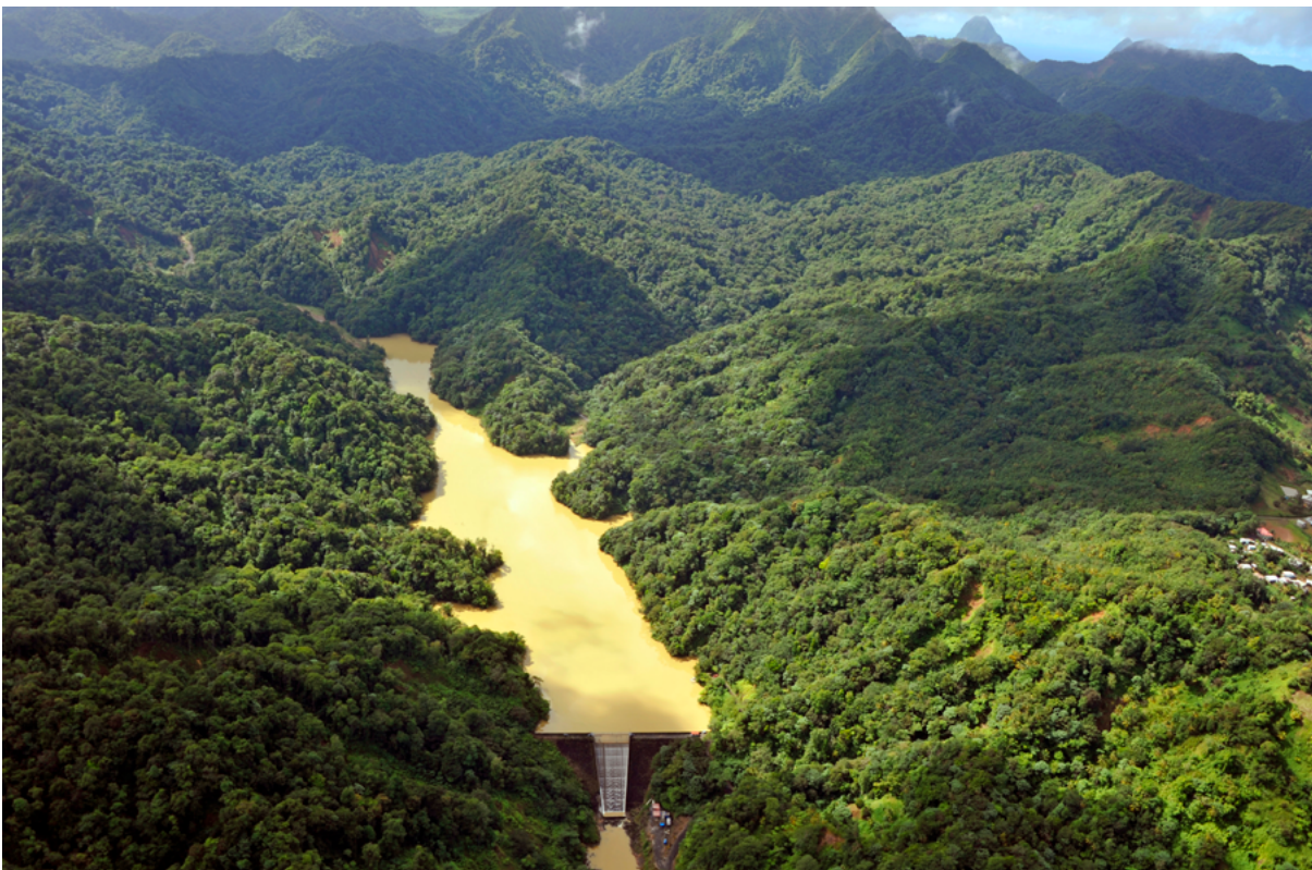
Silt-laden reservoir at John Compton Dam, Saint Lucia. This is the result of heavy rain and landslides. The reservoir is the main water supply for the capital, Castries, and surrounding area. Credit: CARS (Caribbean Aqua-Terrestrial Solutions)
