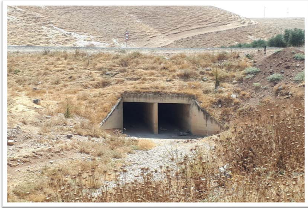
Figure 41: Wadi Yesila 2-Cell Box Culvert
