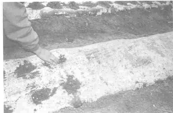
Figure 71. Making holes at seed cracks.
