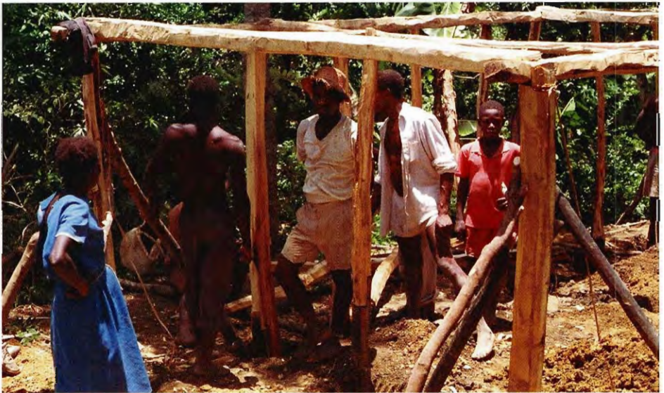
Figure 2.6 C. arborescens is valued as a construction timber used for building houses in Haiti.
