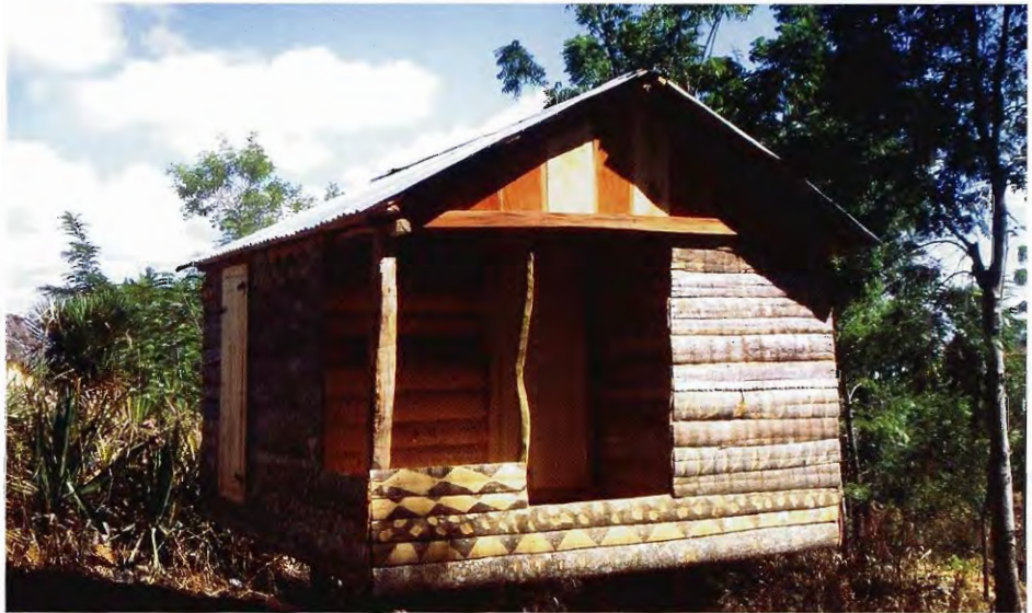
Figure 7.7 R. borinquena is an important source of construction material for granaries and houses, particularly in the Central Plateau.
