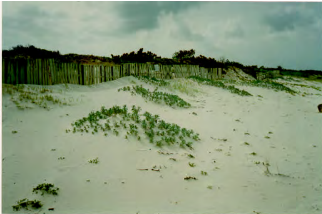
Photograph 7. Sand fence, Shoal Bay, Anguilla, October, 1998, eleven months after installation. Note sand is beginning to accrete in front of the fence.
