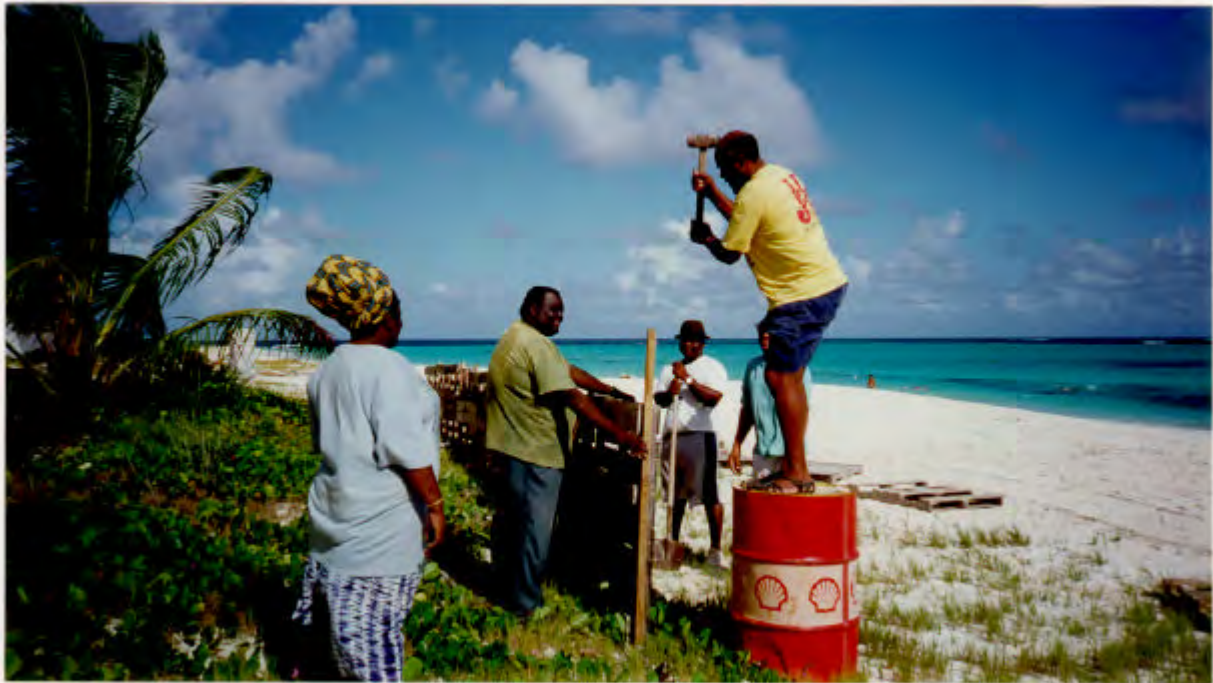
Photograph 6. Sand fence under construction, Shoal Bay, Anguilla, November, 1997.
