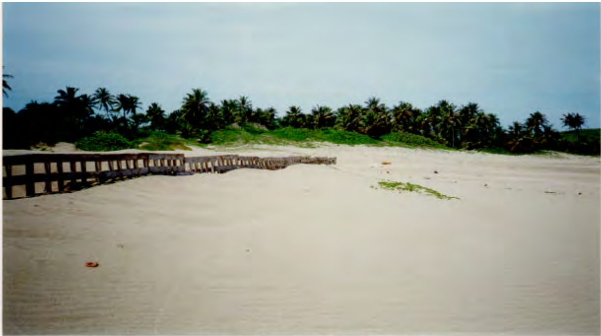
Photograph 5. Sand fence at Barceloneta, Puerto Rico, October, 1997. Note the fence has trapped sand so that the pallets are almost covered.
