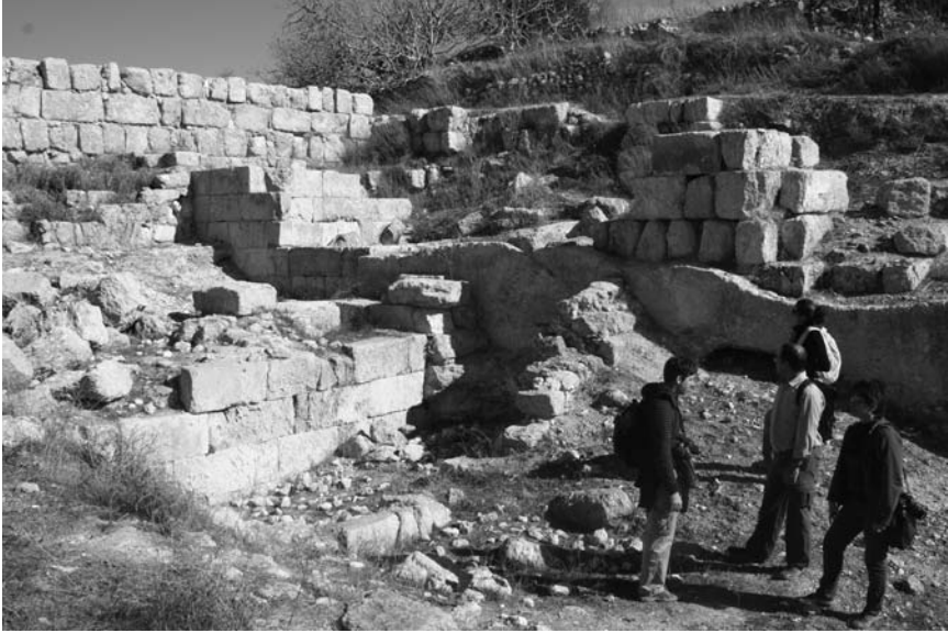
Figure 23. All that can be seen today of the walls of the palace at Samaria. Note the rock scarp and the headers and stretchers building method (wall on upper left side belongs to the temple of Augustus).
