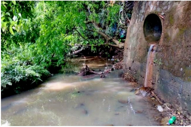
Image 13. Sewage disposal into river through underground tunnel. Kabini sub-catchment from Palvelicham. © Bibin Paul M.
