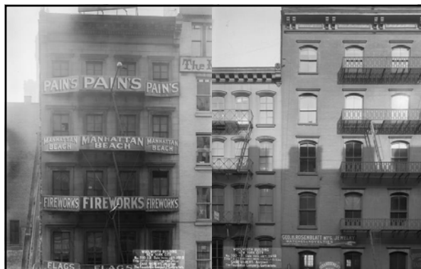
Left: caption: "Woolworth Building, Upper Section of 12 Park Place (Showing Pain's Fireworks), 1910" Right: caption: 229 Broadway, Woolworth Building, West End, Barclay Street Side (Showing Geo. H. Rosenblatt Mfg. Building), 1910"
