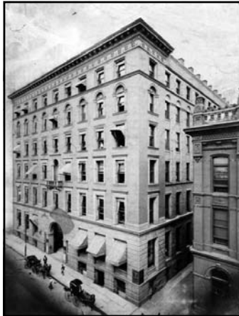
Left: the Endicott Building at 141 East Fourth Street in St. Paul, MN offered Cass Gilbert his first opportunity to employ elements of his beloved Italian Renaissance style on a large scale. The building's elegant design, large size and high standard of construction made it the premier office building in St. Paul . The exterior features a granite base, brownstone facing (on the first floor) and pressed brick above. The cornice is made of terra cotta. An important feature of the Endicott Building is the presence of an arcade of shops on street level - a forward-looking design (Arcades were incorporated in a number of Gilbert's later office buildings, including Woolworth ). The Arcade is lavishly detailed in exotic colored marbles, stained glass and stone mosaic floor tile.
