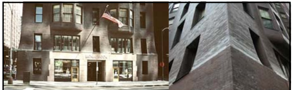
"...a new difficulty arose: the brick walls at the base became thicker than ever, and their cost was enormous; their weight, too, was excessive for the foundations, and it was soon found that the ground space they occupied caused great loss to owners. So thick, in fact, were the walls at that time that if an owner built on a narrow lot he had little more than an entrance hallway between the side walls on the ground floor..."
