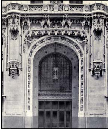
An elaborately carved stone balcony and related ornamental projections, in collaboration with the arch and bays, form a triumphal arch. The motif of the stone carvings are Gothic-inspired. The balcony includes narrow panels with shields separating wide panels of Gothic tracery over the entrance and wide panels with stylized flowers over the flanking bays. The center panel supports a large eagle holding a shield at its breast. From either side of the entrance arch, an elaborately carved niche with Gothic tracery descends, culminating with a carved coiled serpent at its base. Similar deep relief Gothic tracery (with fanciful grotesques) link the balcony with the arches of the entry and its flanking bays. A depressed arch outlined with a course of trefoil tracery frames the tudor-arch entrance. 421
