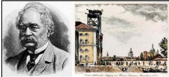
In April 1880, Werner von Siemens (left) demonstrated the first electric powered elevator at the "Mannheim Pfalzgau Trade & Agricultural Exhibition" (right). With a motor mounted on the bottom of the cab, Siemens' electric elevator used a gearing system to climb wall shafts fitted with racks. Although novel, this electric elevator was still too crude to compete with the existing steam-driven, hydraulic elevator technology. Intended simply as an illustration of the broad applicability of his pioneering work in DC traction motors, Siemens had little interest in pursuing the electric elevator further. Instead, Siemens focused on large projects, such as electric trains and electric power systems.
