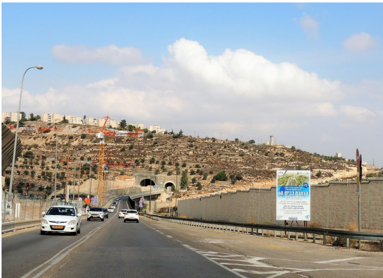
Digging another tunnel to double the Tunnels Road (Bethlehem Bypass), November 2020.
