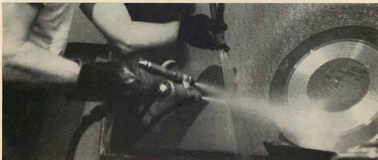
A thin layer of silver is deposited on the lacquer by spraying the disc simultaneously with a silver solution and a reducing agent.
