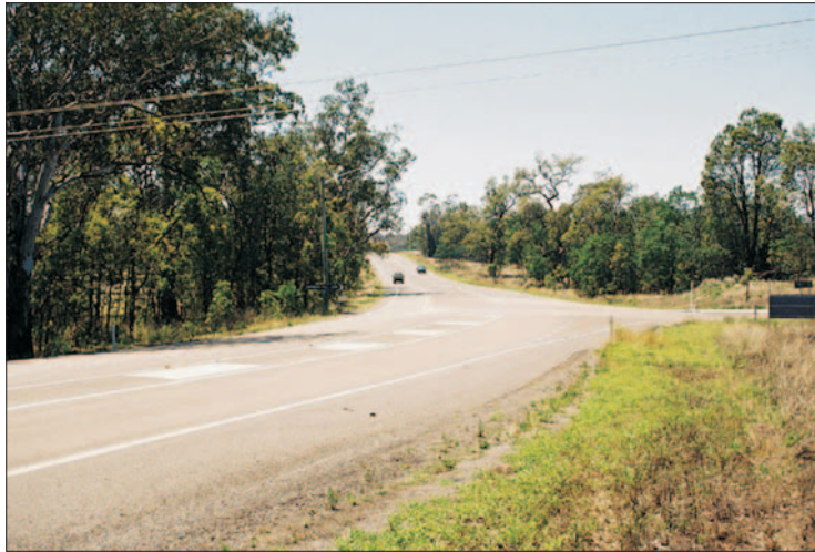
Plate M-5 Golden Highway at Wambo Access Road Intersection - View Looking East
