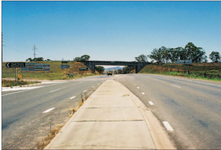
Plate M-1 Putty Road / Golden Highway Showing the Mount Thorley Road Overpass
