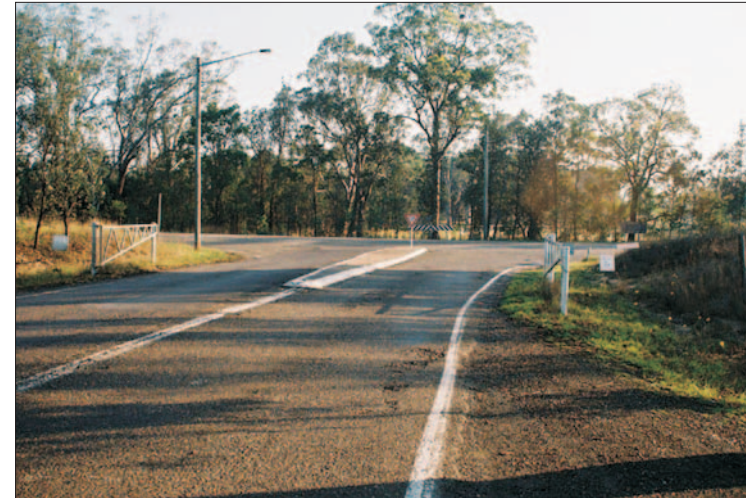
Plate M-6 Wambo Access Road Looking Towards the Golden Highway Intersection
