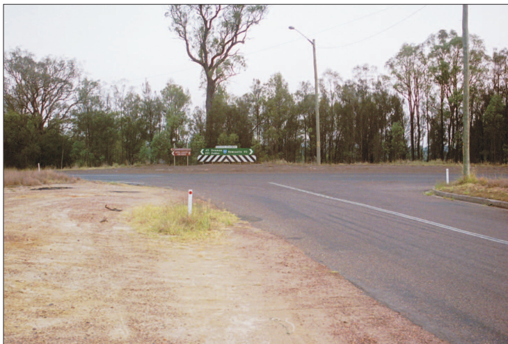
Plate M-3 Wallaby Scrub Road / Golden Highway Intersection - View from Wallaby Scrub Road
