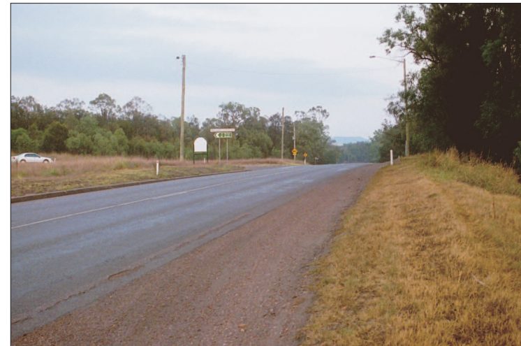
Plate M-4 Wallaby Scrub Road / Golden Highway Intersection - View Looking West on the Golden Highway
