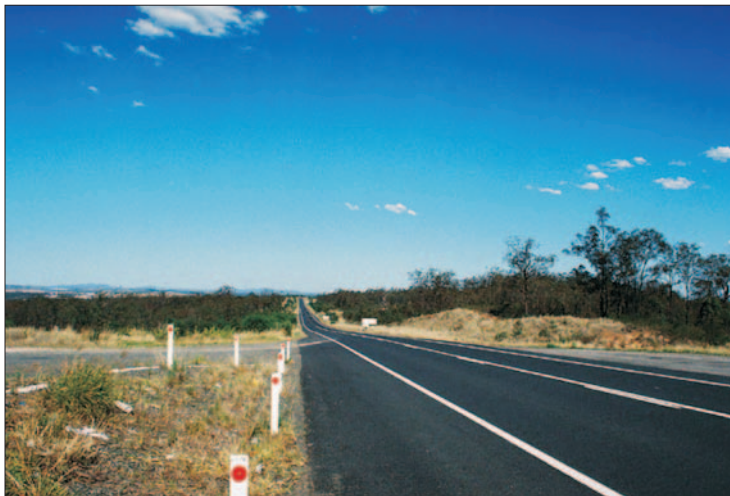
Plate M-7 Golden Highway North of the Project Looking East
