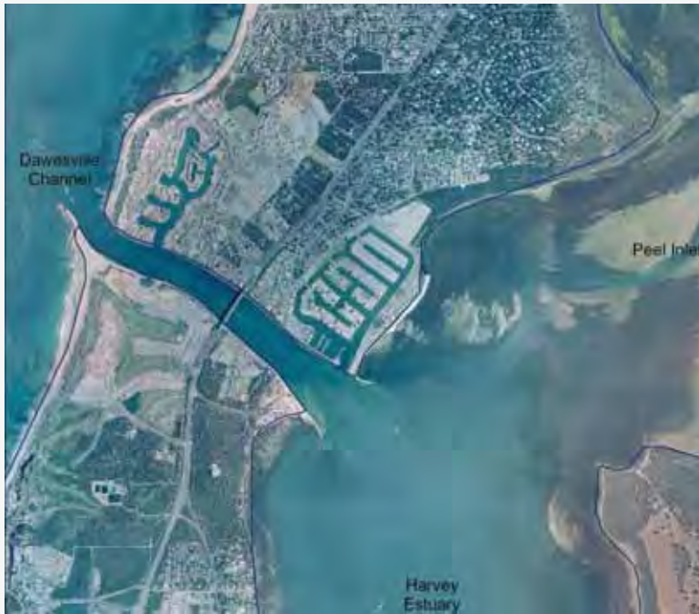
Figure 35: Aerial image of the Dawesville Channel.
