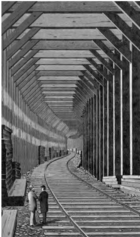
Figure 37: Snow shed on the Central Pacific Railroad.
