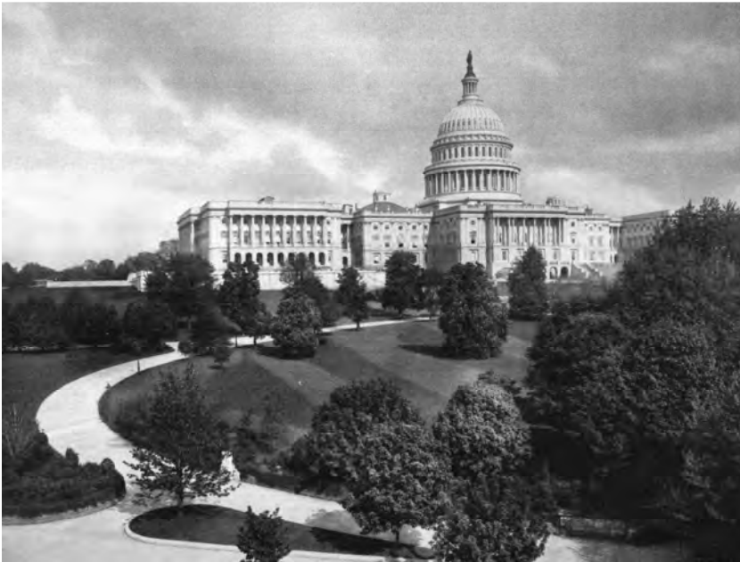
Figure 10: West front view of the Capitol.
