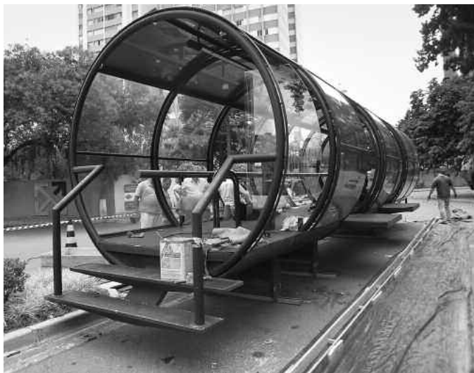
A bus stop shelter under construction in Curitiba, Brazil
