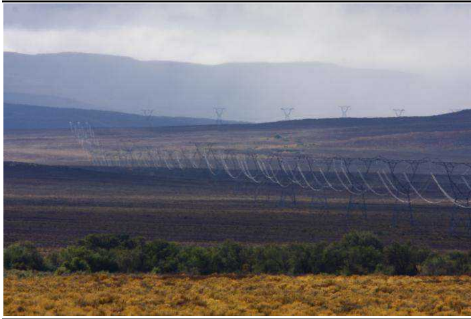
Figure 5.12 Acacia karoo woodland along the bed of the Groot River, with the Bachus-Droërvier 400 kV transmission line in the background
