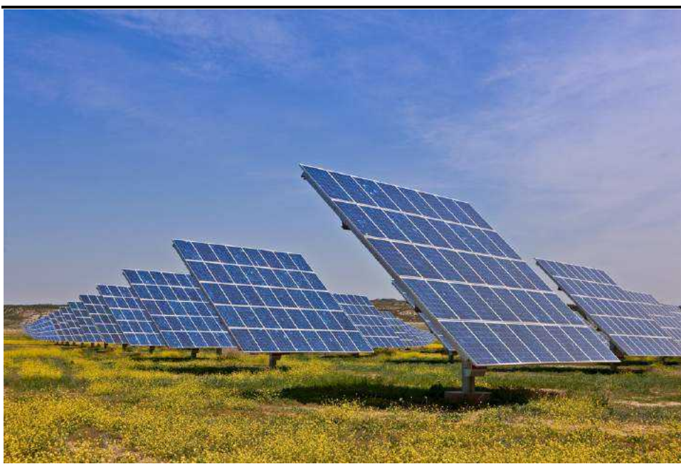
Figure 4.3 Typical PV Panel Arrays
