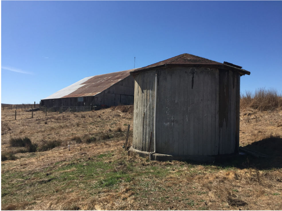
11 - Existing water tank
