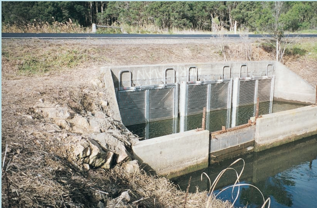
Aluminium screens to restrict carp movement into Macleods Morass. Source: A. Brumley, East Gippsland Institute of TAFE.
