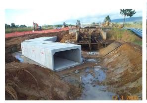
Figure 6: Construction of box culvert outlet.
