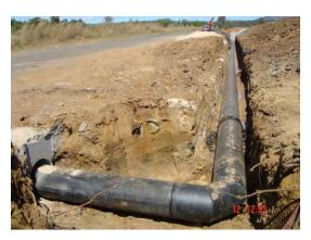
**Figure 8:** Filtrate pipeline from fish screen at road crossing.
