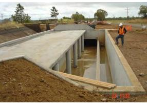
**Figure 7:** Completed concrete screen structure before screens installed.
