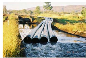
Figure 5: Bypass temporary supply pipes
