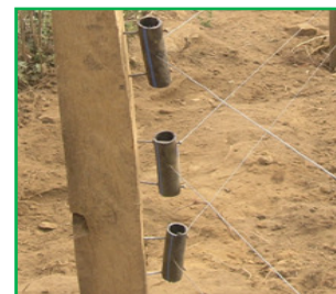
HDPE Pipe pieces used as Insulators
