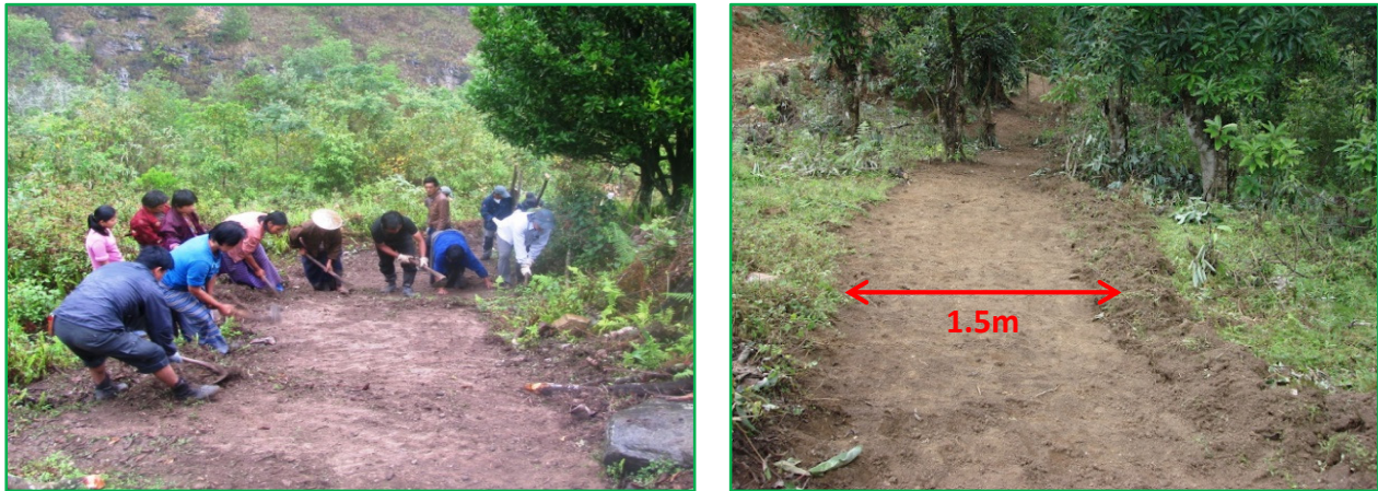
Figure 7. Clearing and surfacing fence line
