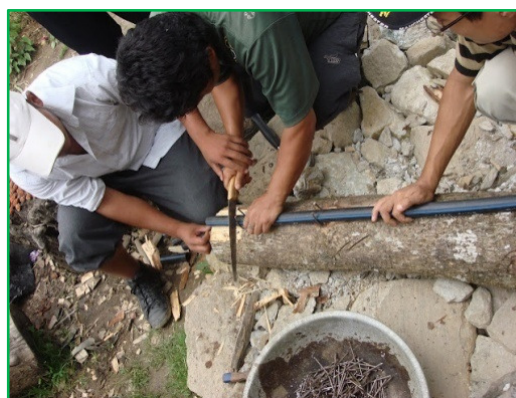
Figure 6B. Preparing HDPE pipe insulators
