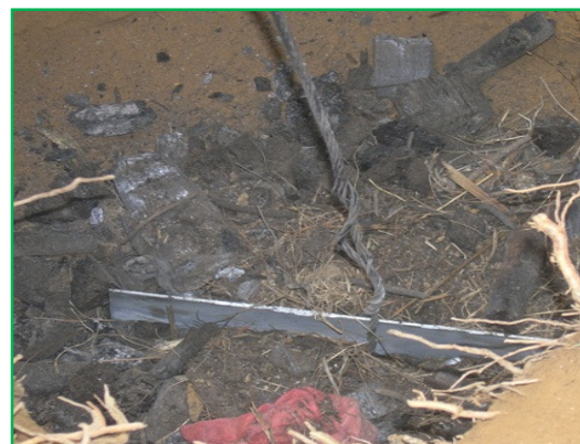
Figure 23B. GI earth plate placed vertically in the pit
