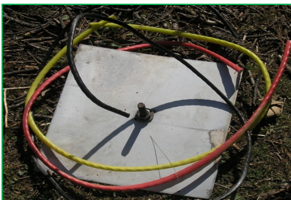
Figure 23A. GI earth plate
