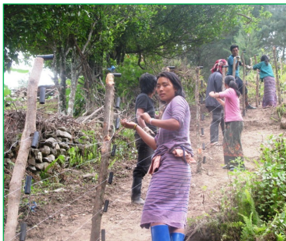
Figure 15: Fixing GI wire
