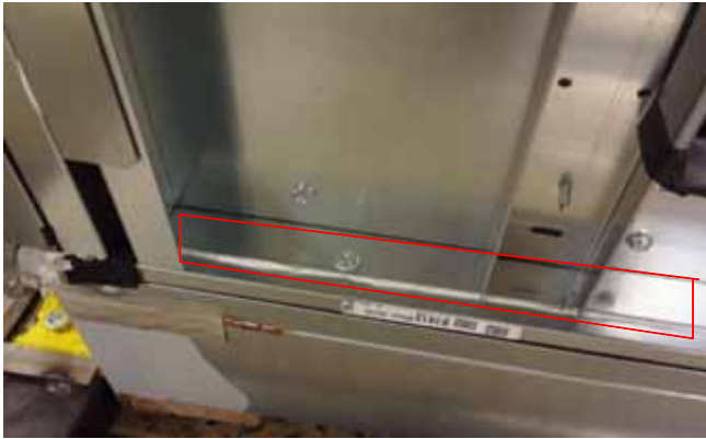
Figure 11. COU panel and filter racks
