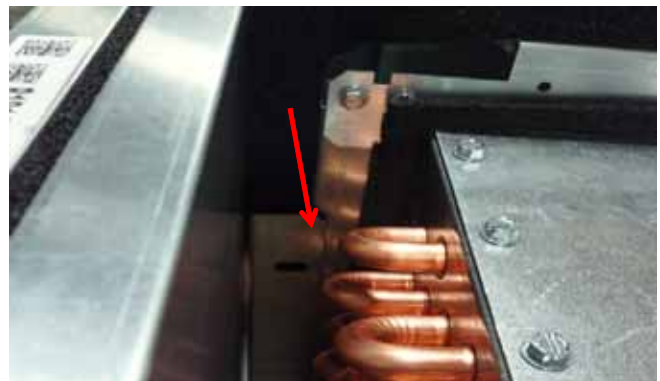
Figure 15. Coil installation
