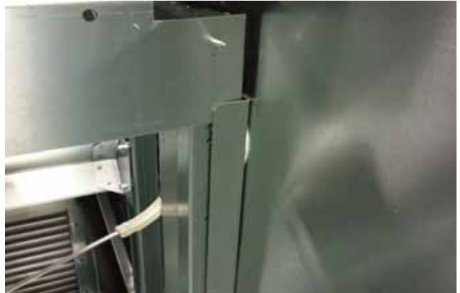
Figure 20. Filter frame removal
