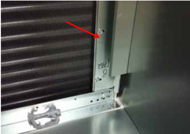
Figure 16. Coil blockoffs
