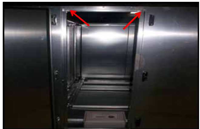
Figure 5. Door header and jambs
