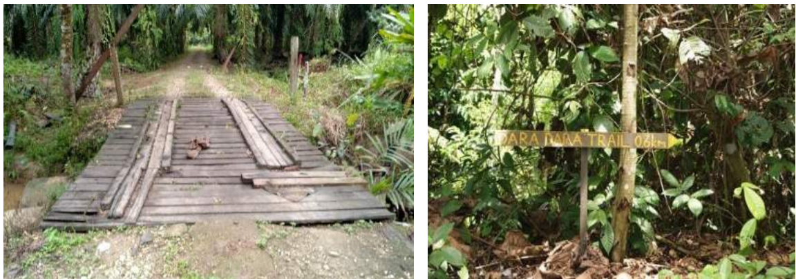
Plate 13: Other infrastructure within the Pin-Supu FR: A. wooden bridge to access field checking station; and B. an example of the many nature trails for recreation facilities.
