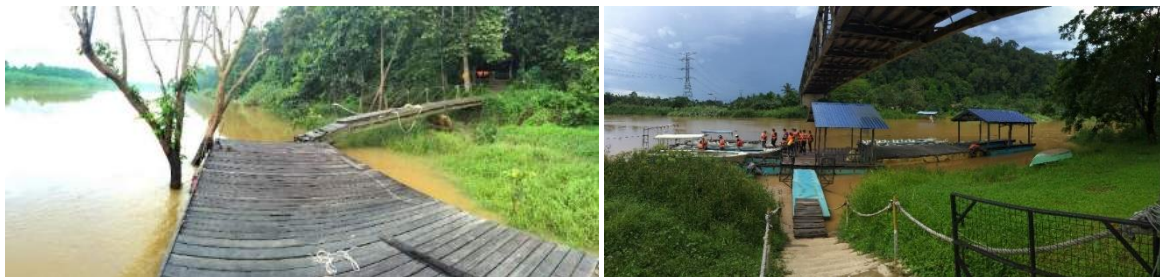
Plate 11: Openwork timber jetties that consist of a platform and bridge in the area.
