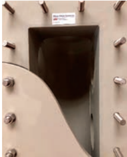
Bolted cover plates
