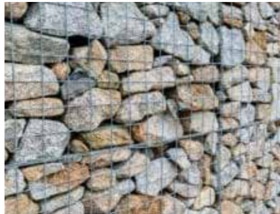
W1 - Gabion Wall - Local Stone
