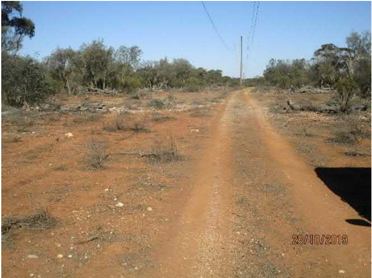
Plate 3-58: Site 10c, Clearance of Mallee either side of the track up to 10m back (facing east)
