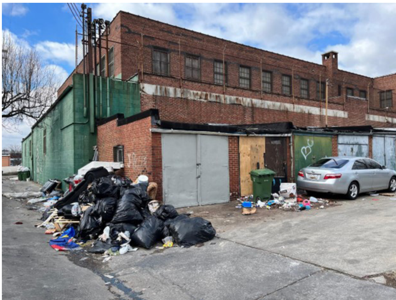
Illegal dumping behind former Hathway's Furniture building, 3501 Pulaski Highway (January 18, 2022)
