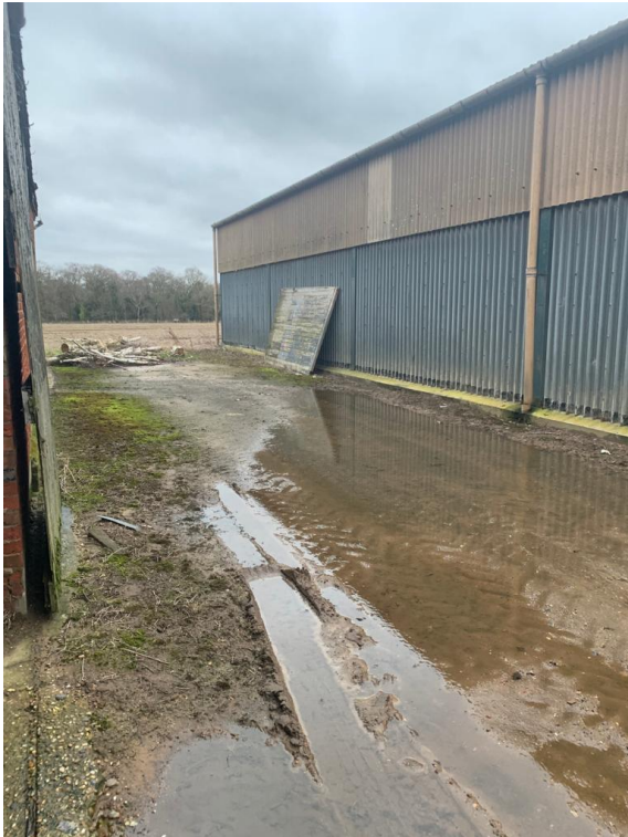
Photo 5: Eastern side of building, with bare ground and hard standing
