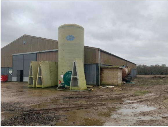
Photo 1: North western corner of building, with hard standing extending north
