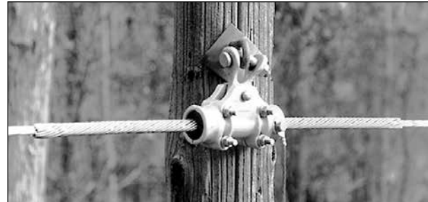
FIBERLIGN Cushion Clamp installed
