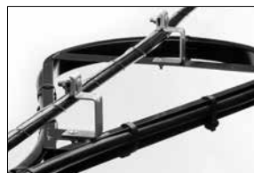
FISA "M" Bracket Installed Messenger Application
