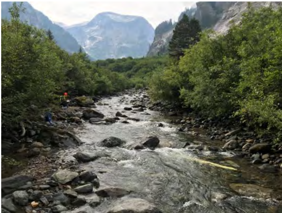
Note exposed pipeline (yellow) in stream.
